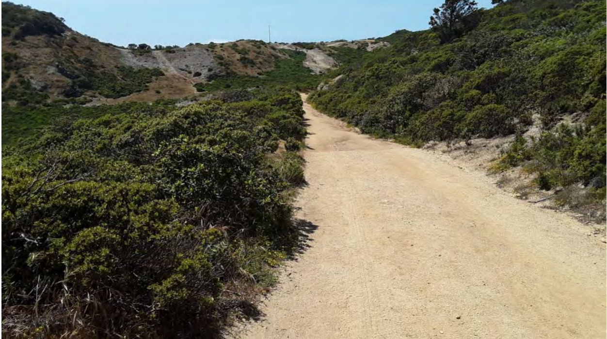
Figure 17: View south of Station 184 at mile 3.5 where the 10-foot roadway would need to be widened to 20 feet to meet the requirements of the proposed fire turnout. This would require extensive vegetation removal.
