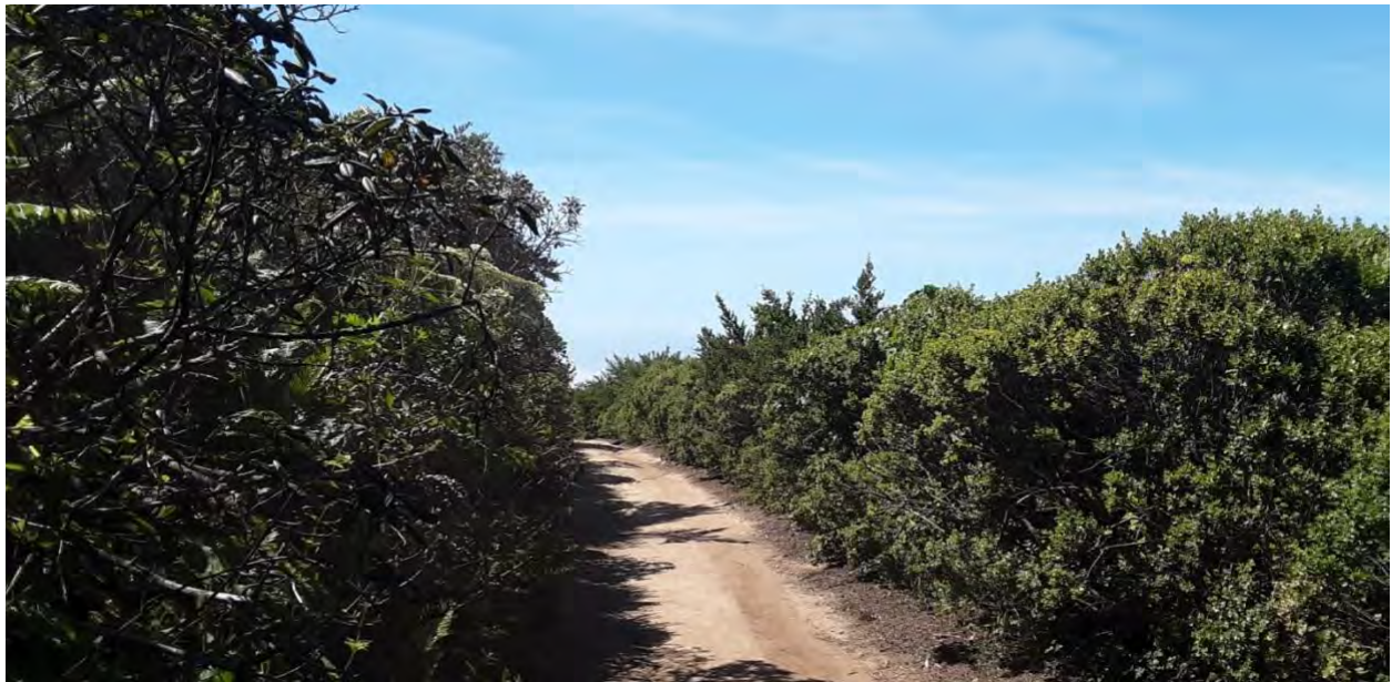
Figure 12: Facing west, view of the access road narrowing to ~8 feet in width above Station 136+00 where many areas are lined with dense coastal scrub. The removal of 4 feet of vegetation from the roadway to meet the 12-foot width requirement for straight-aways and the removal of 7 feet of vegetation along road curves to meet the 15-foot width corner requirement will cause an impact.
