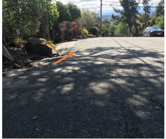
PHOTO 2: Drainage swale at the top of the driveway
