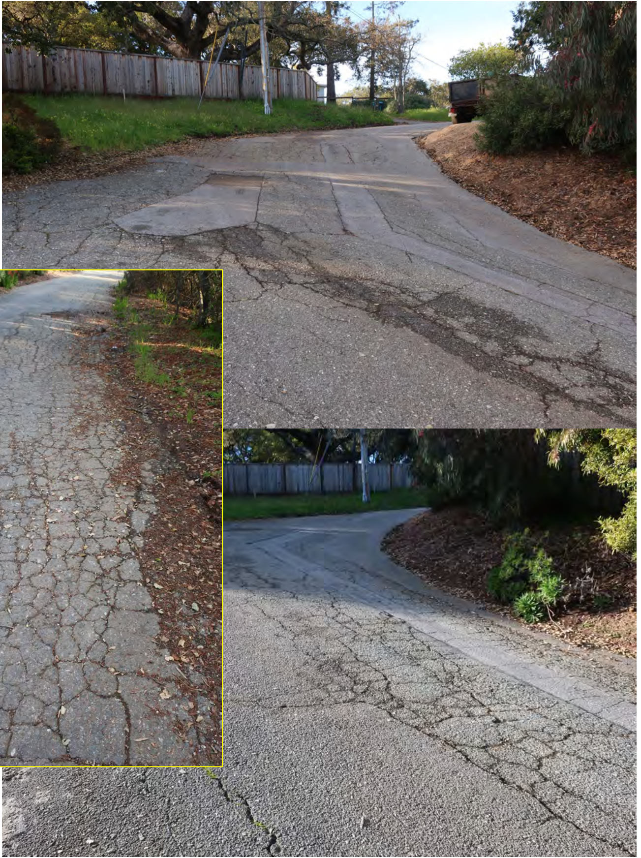
Figure 5. Photos checked and patched asphalt indicating underlying water along Loma Rd, San Mateo County, CA. Photos taken on March 2, 2023.
