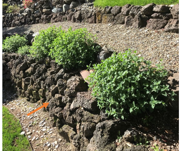
PHOTO 5: Terraced and drained retaining walls
